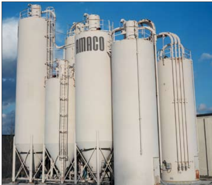
Silos photo courtesy of Ginny Taylor Rosner, Images Custom Photography.
